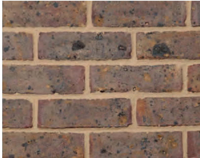
01 Brown multi brickwork
