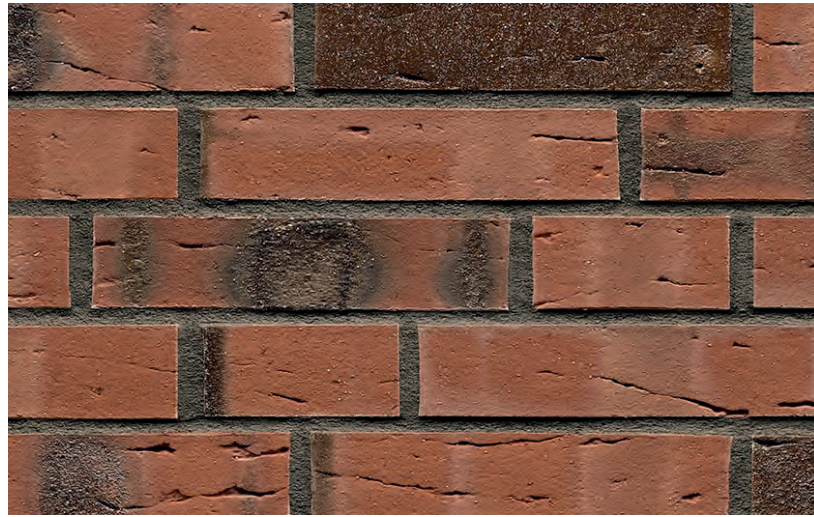
01 Earthy red multi stock waterstruck brickwork
